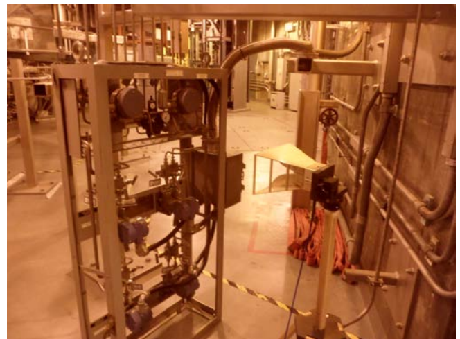
Figure 3. Mapping Location in Nine Mile Point Unit 1 Reactor Building
